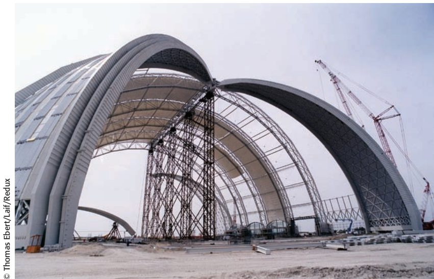
The equilibrium of structural components such as these shell-like panels is an issue both during and after construction. This structure will be used to house airships.
