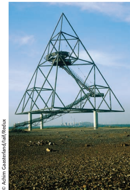
This space truss is used to support observation equipment in Bottrop, Germany.
